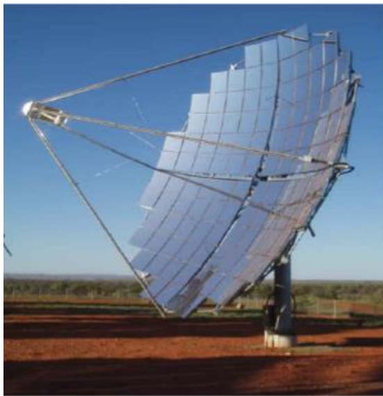
Figure 7: Concentrated PV systems [32].
